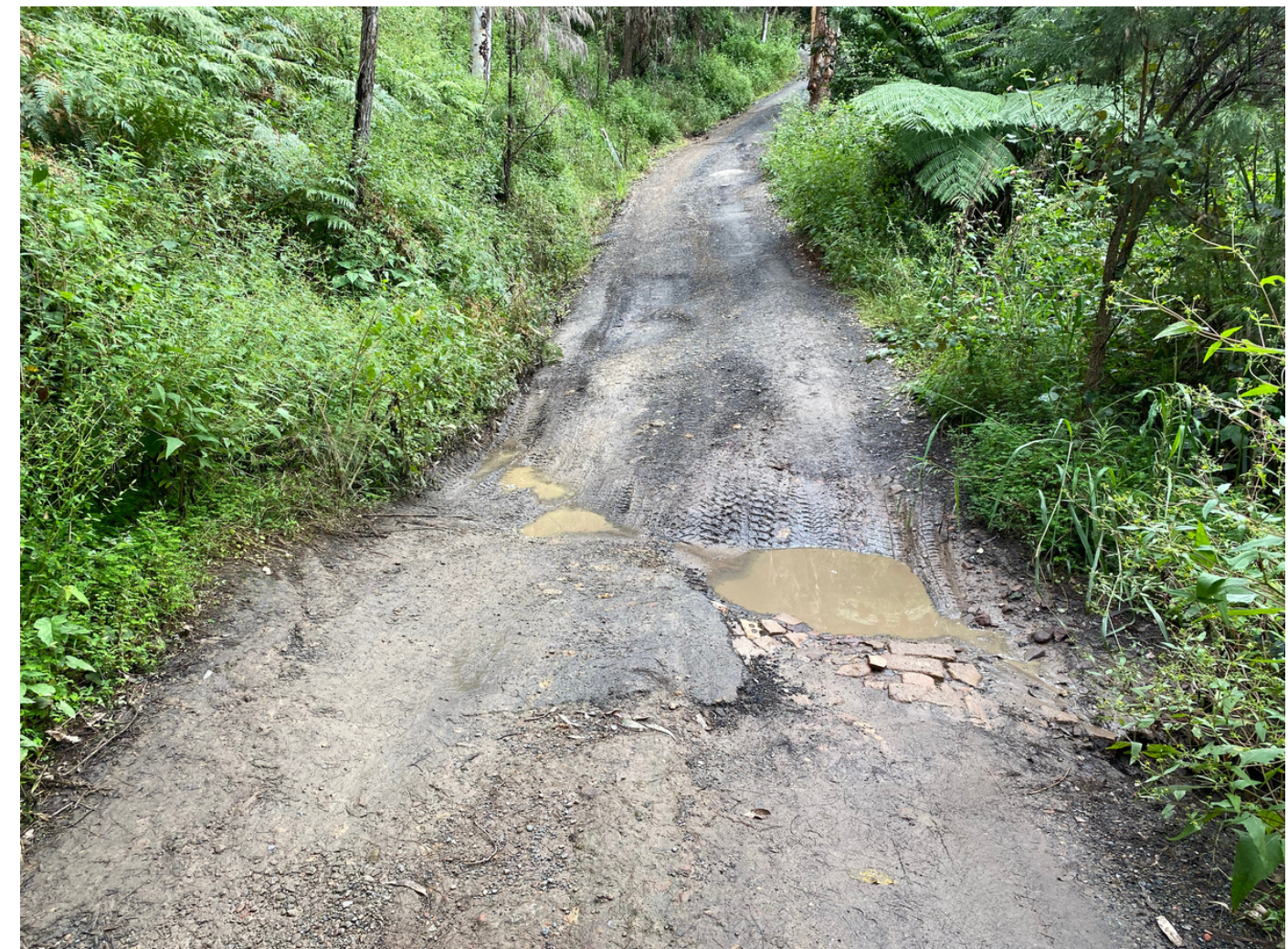
Photos showing rain damage on Scotland Island Roads courtesy Shane O'Neill
