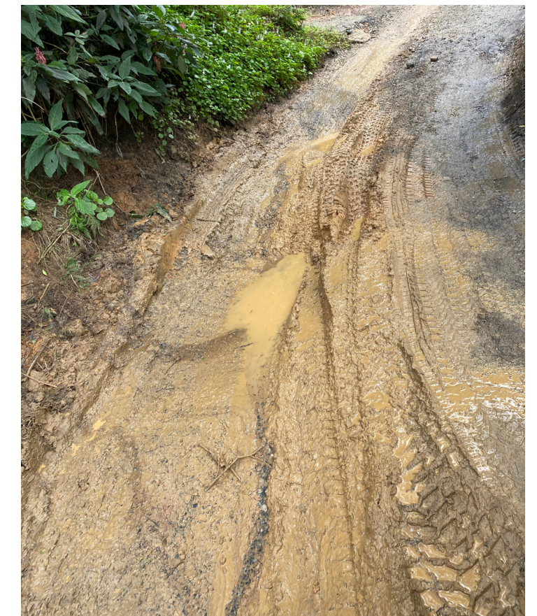
Photos showing rain damage on Scotland Island Roads courtesy Shane O'Neill
